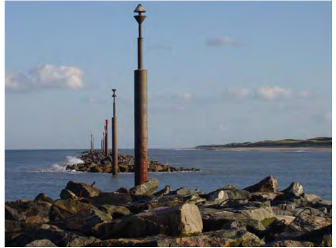
A coastal protection reef at Sea Palling. Such hard sea defences are likely to alter the sediment supply to beaches and sandbanks further along the coast.
