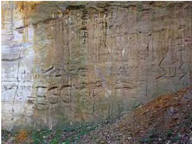
Graffiti damage at Dersingham Sand Pit, part of a SSSI and the type-site of the Lower Cretaceous Dersingham Formation.
