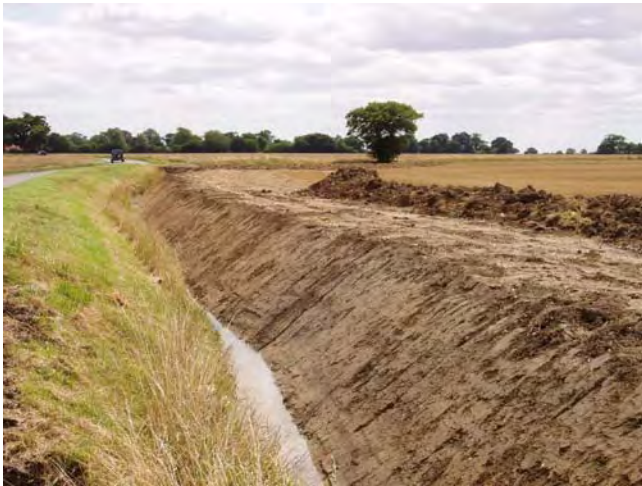
Heath Farm, Banham, Deep ditches are essential to drain the stagnogley soils of the till plateau of south and central Norfolk. Waterlogging means early harvesting of sugar beet in wet years and autumn sowing of winter cereals.
