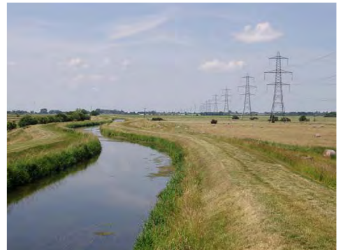
The River Nar at Middleton. The river is artificially embanked and is perched over two metres above its floodplain. It is now prone to siltation and disconnected from a formative relationship with its floodplain.
