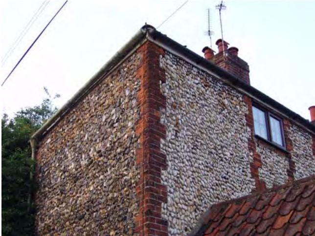
Cottage walls at Thorpe St Andrew, built from contrasting panels of knapped (broken) and nodular flint.
