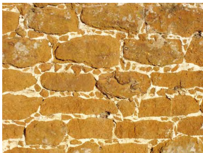
A Carstone wall at Snettisham. Carstone is a useful building stone which tends to harden with age. It is also quarried to supply hardcore for roads.
